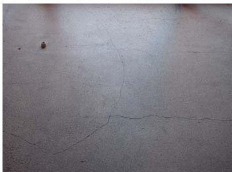
PvI-02-FI-07 Internal floor - Floor Cracking - Variation of humidity and temperature
