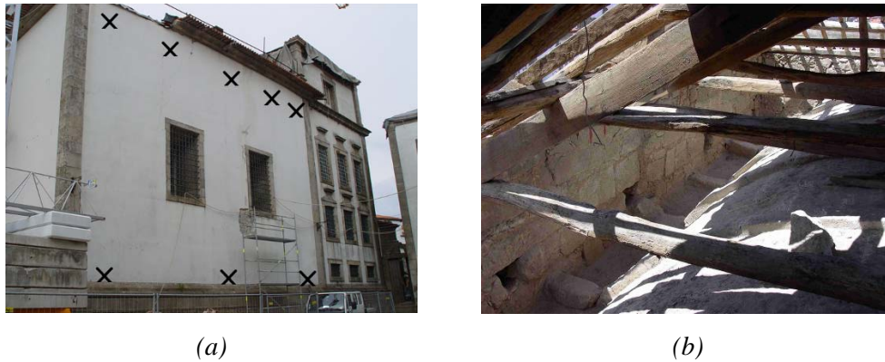
Figure 17. Infill removal: (a) location of topographic targets for monitoring; (b) aspect of the cleaned vault.
