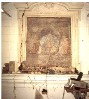
Figure 34: The tested wall at the Brera Palace.
