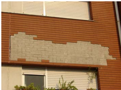
PE-02-DE-03 External wall - Covering Degradation - Blistering
