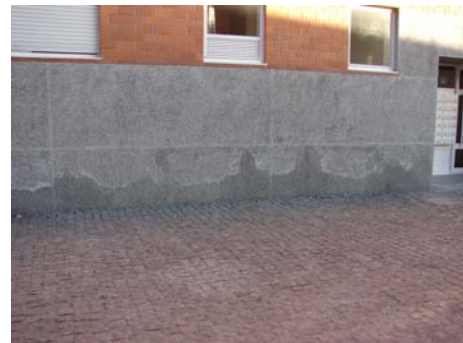
PE-02-HU-01 External wall - Covering Humidity - Ascensional from soil
