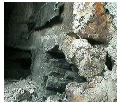
Figure 36: Borehole inspection of the cavity at the Brera Palace.
