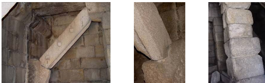
Figure 8: Deficient structural system to support the bell stone level floor.
