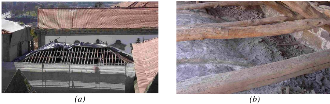
Figure 14. Roof of Saint Vincent Chapel: (a) aspect of restoration works; (b) aspect of vault infill with rubble.
