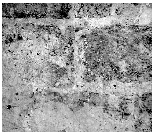
Figure 16: Regular stone-block masonry and regular stone-block masonry with "incoccio" in the S. Nicolò Church.
