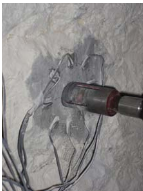
Fig. 7 “Hole Drilling test”
