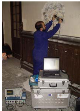
Fig. 8 “Impact echo test on a masonry wall”
