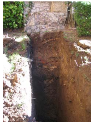
Fig. 19 "Soil Pit for recognition the foundation of South facade wall"
