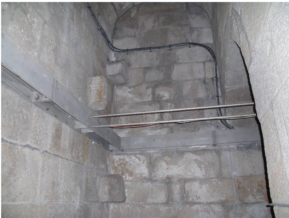
Fig. 3 General sight of the reinforcement system
